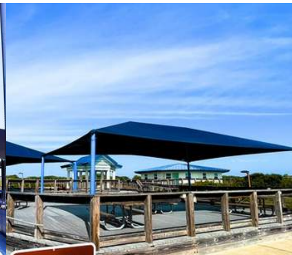
Hip Shade Structure
